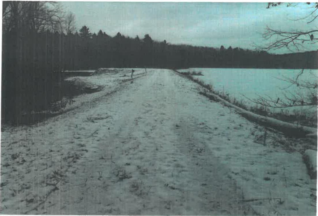
Photo 3 Dam ID# 243-1430 Martin Dunham Reservoir Dam 01/05/2024 Left auxiliary spillway closure embankment
