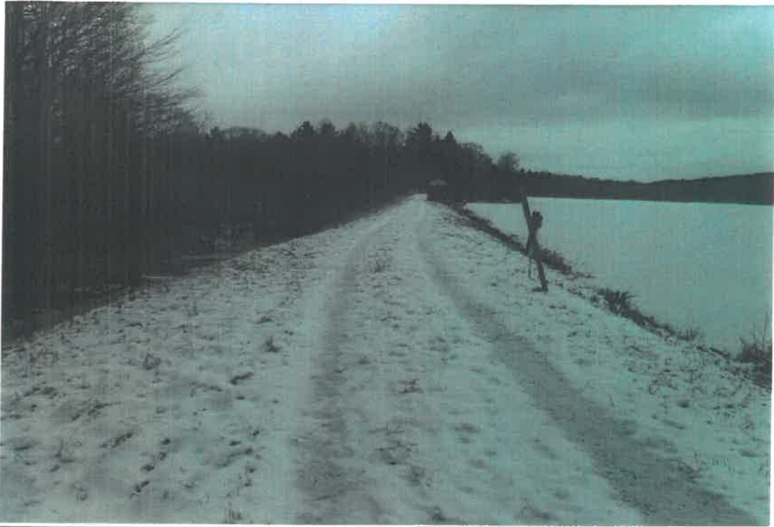
Photo 1 Dam ID# 243-1430 Martin Dunham Reservoir Dam 01/05/2024 Dam crest
