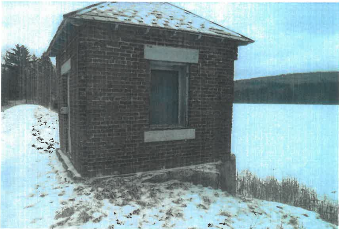
Photo 2 Dam ID# 243-1430 Martin Dunham Reservoir Dam 01/05/2024 Valve house
