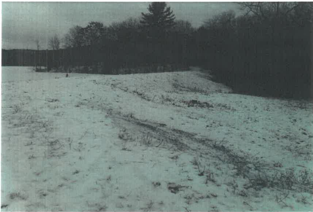
Photo 8 Dam ID# 243-1430 Martin Dunham Reservoir Dam 01/05/2024 Left auxiliary spillway closure embankment
