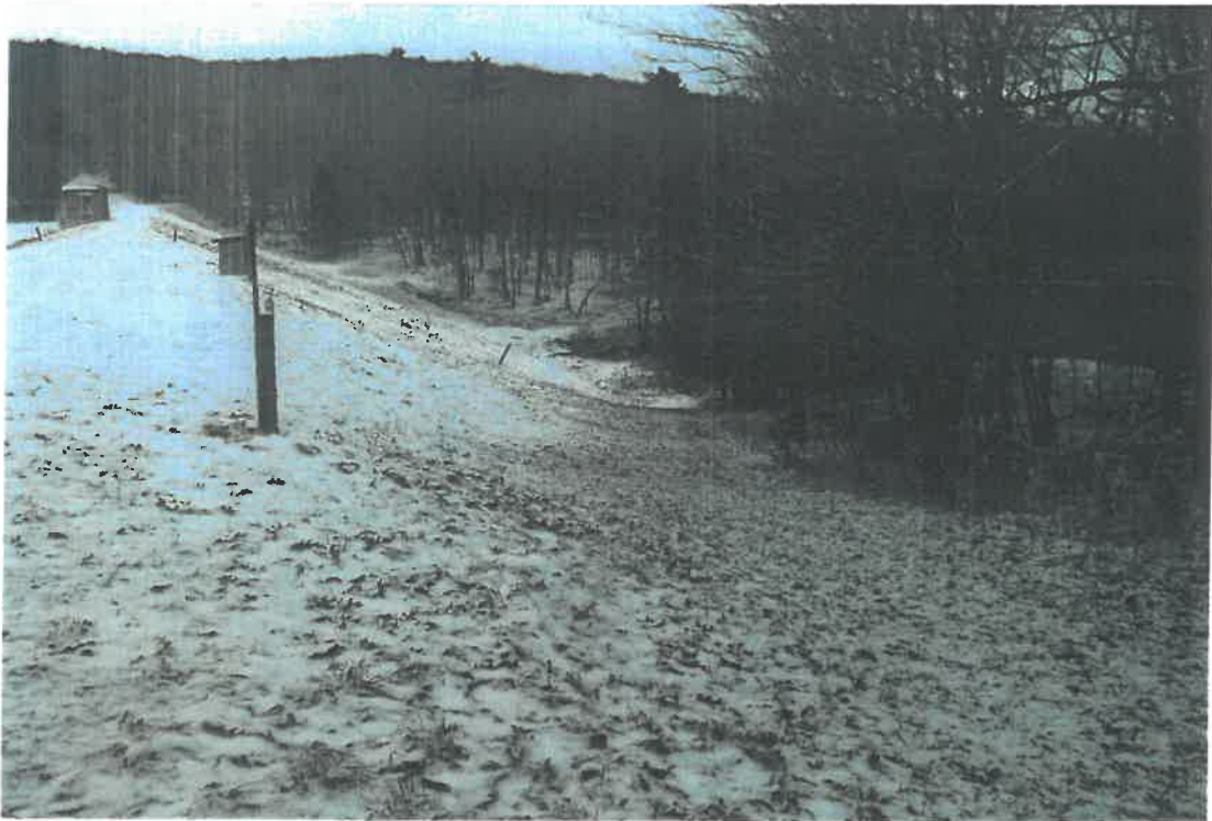
Photo 9 Dam ID# 243-1430 Martin Dunham Reservoir Dam 01/05/2024 Downstream face of the dam
