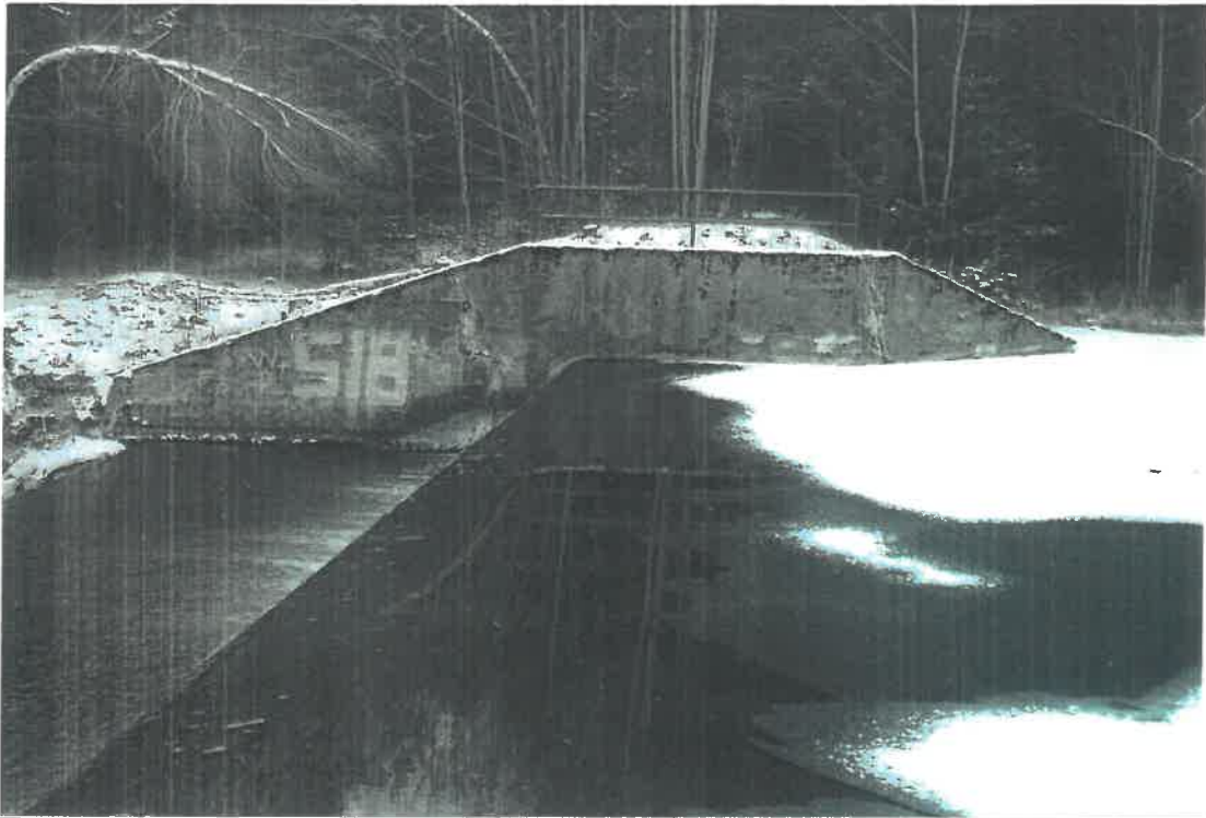
Photo 7 Dam ID# 243-1430 Martin Dunham Reservoir Dam 01/05/2024 Right spillway wall
