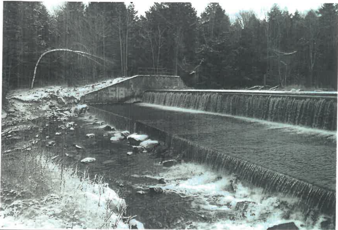
Photo 5 Dam ID# 243-1430 Martin Dunham Reservoir Dam 01/05/2024 Spillway
