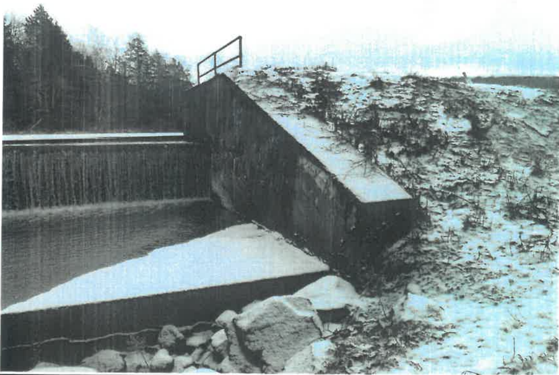
Photo 6 Dam ID# 243-1430 Martin Dunham Reservoir Dam 01/05/2024 Left spillway wall
